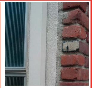
Above you can see an example of an exterior window joint. It is important to check window joints in order to insure that water is not making its way indoors through any weaknesses in the joints.
